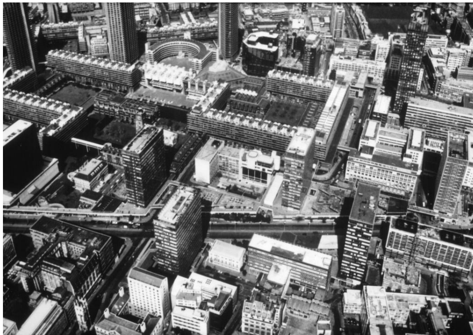
Category 5: Dense urban areas and city centres (e.g. buildings of four-stories or higher) with a plan area density of greater than about 20%.
